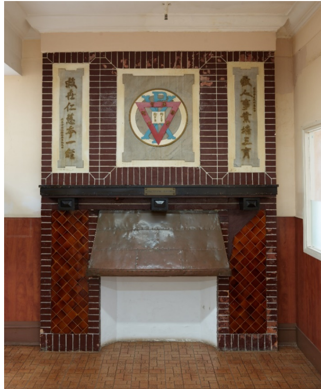
The fireplace on ground floor. The emblem of YMCA and couplets backed with marble plate and slabs are on top of the mantle.
